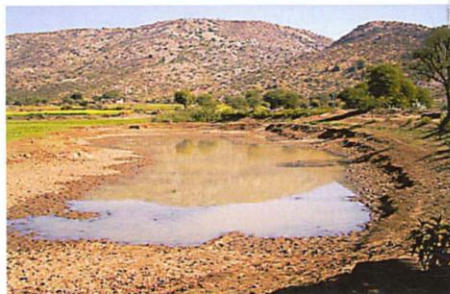
In Rajasthan, johads or earthen dams have been used for thousands of years to conserve the meagre rainwater for drinking and irrigation.
